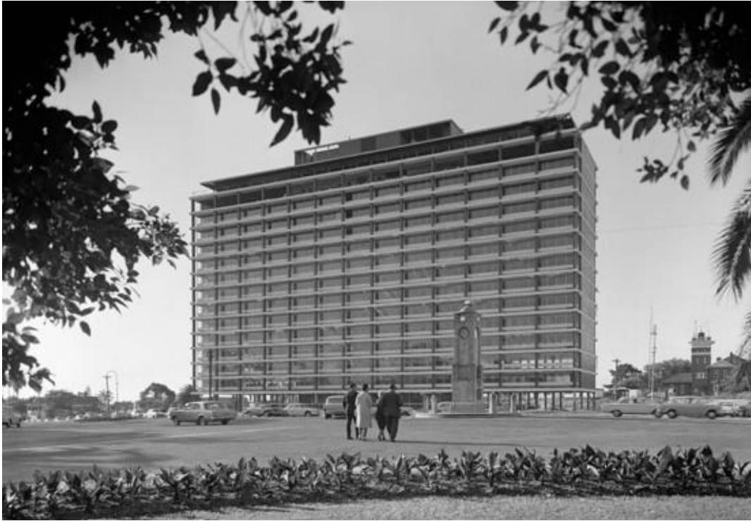
Fritz Kos' 1965 photo of the nearly finished Dumas House at West Perth (SLWA 340709PD).
